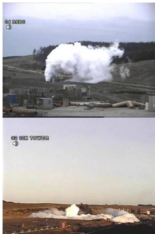
Figure 8.3: Vertical discharge versus 'blanket' formation
