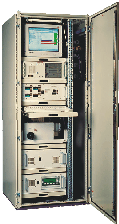
Figure 27: The GASMET CEMS used at LYPP to measure various compounds and emissions
