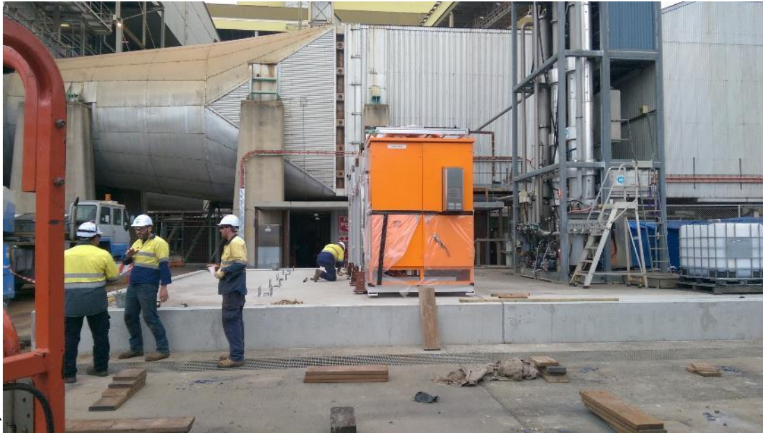
Figure 15 First module in place and being levelled
