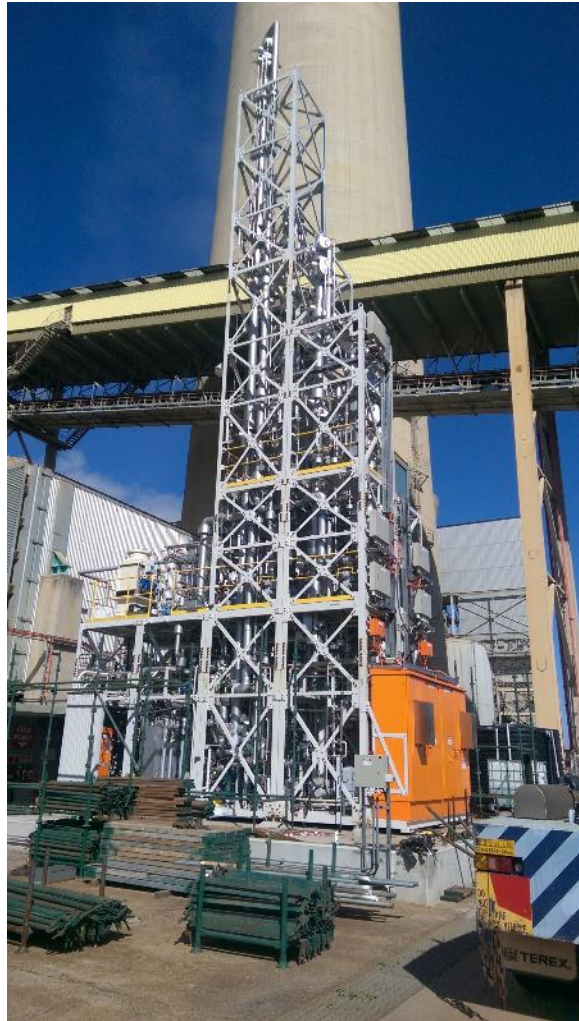
Figure 24 Mechanical installation complete
