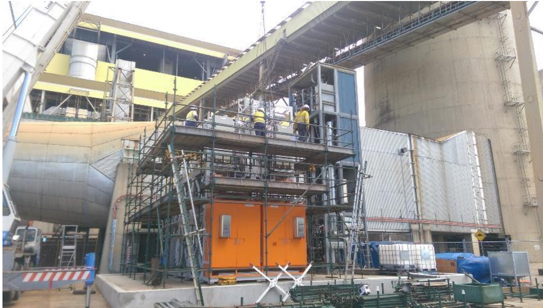
Figure 19 Scaffolding construction for higher level modules. Fifth module in place
