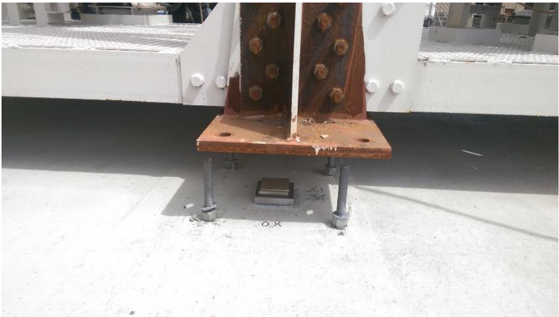
Figure 11 First attempt at installing the module
