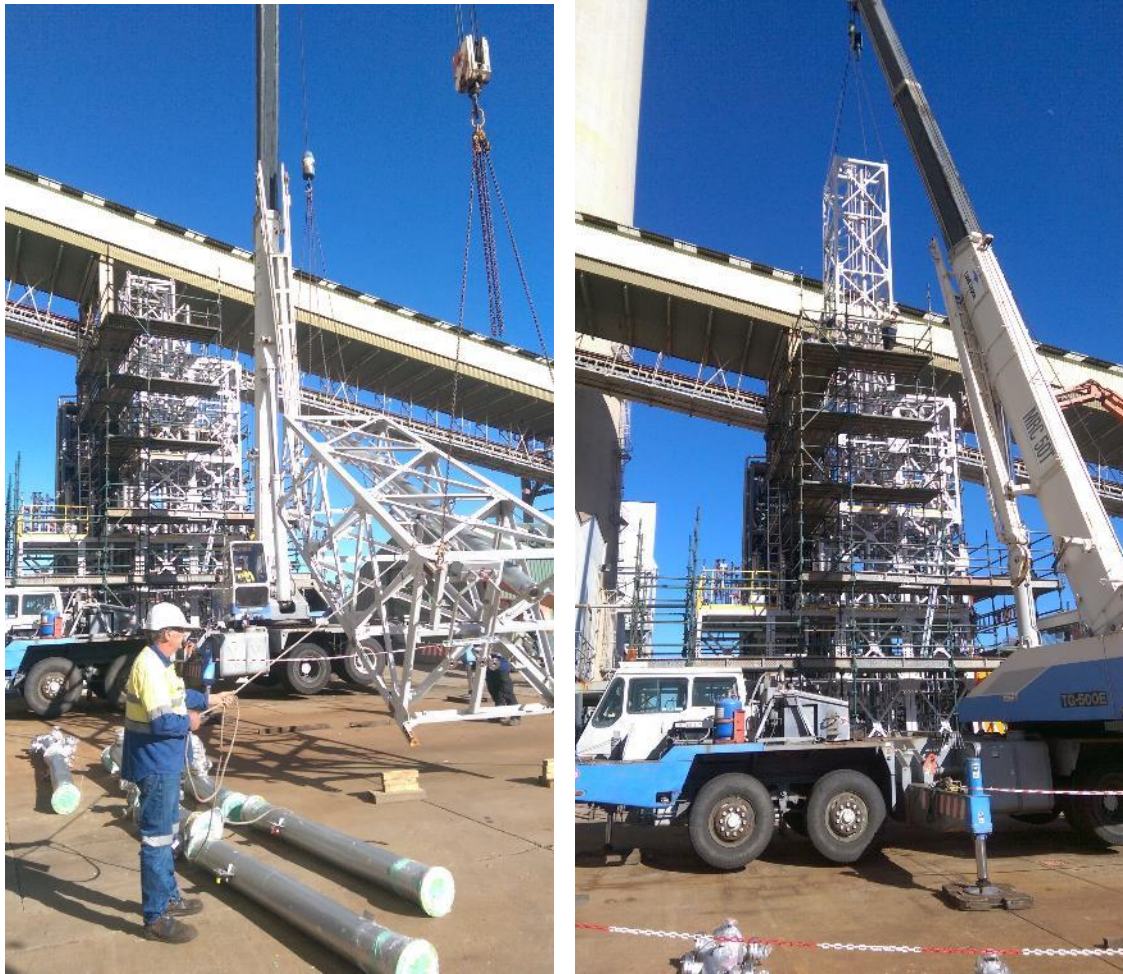
Figure 23 Final module lift using two cranes and positioning to complete structure.
