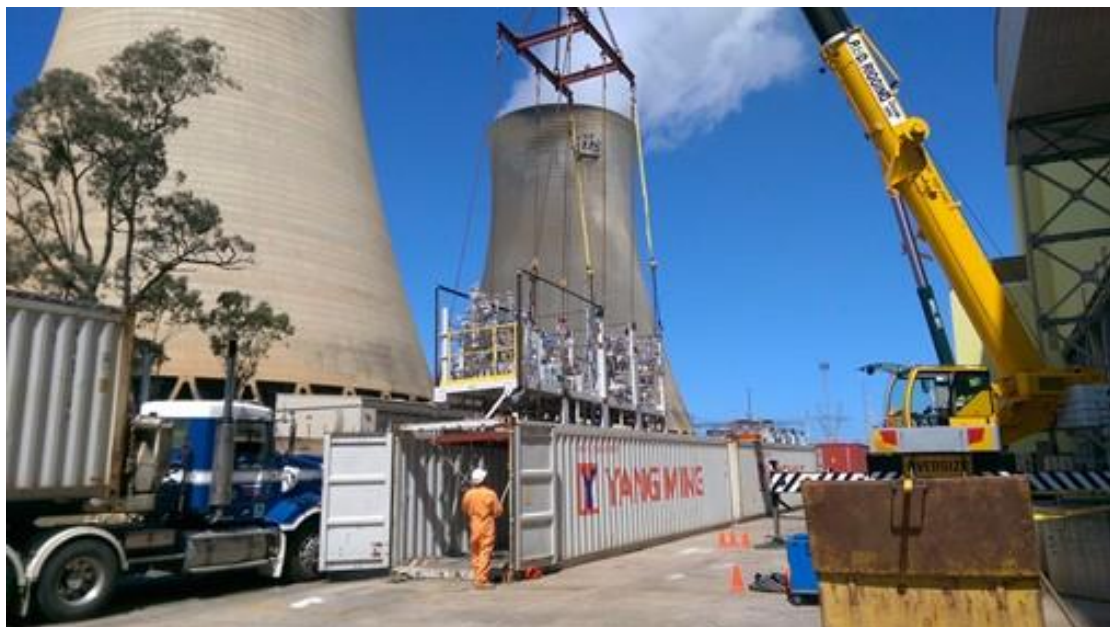
Figure 10 Unpacking of delivery containers at laydown area next to Unit 4.
