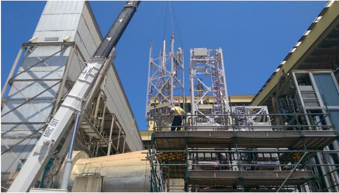
Figure 21 Seventh module installation
