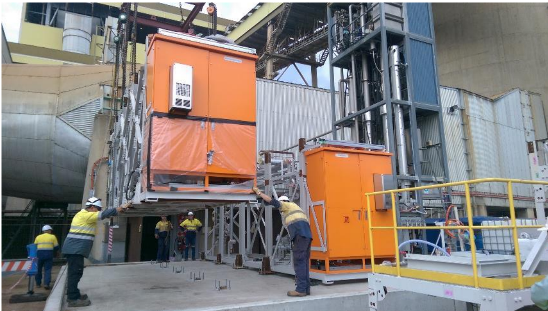
Figure 16 Second module installation
