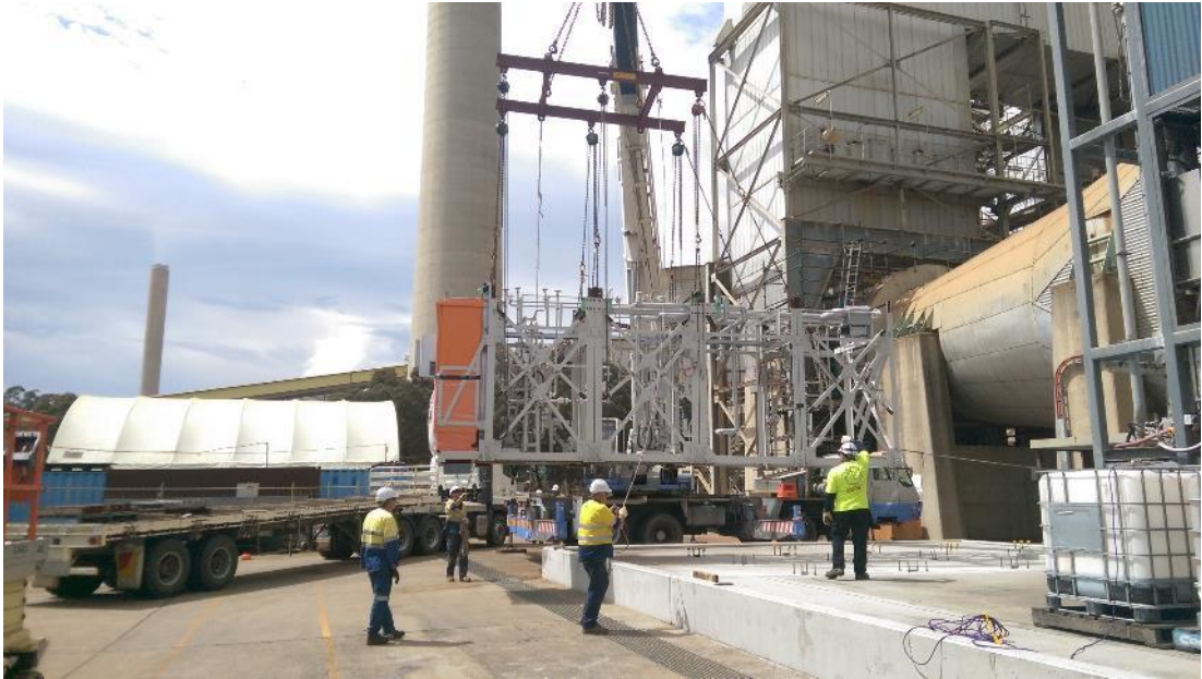
Figure 11 First attempt at installing the module
