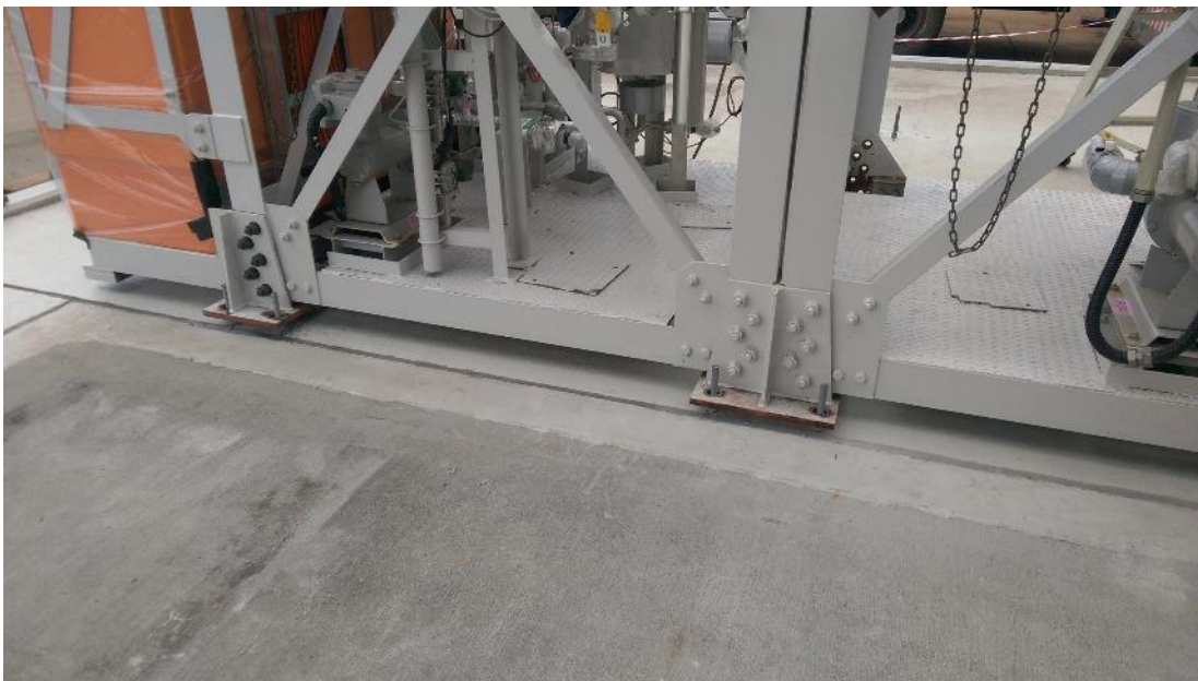
Figure 14 Good fitment of modules after support bracket modifications
