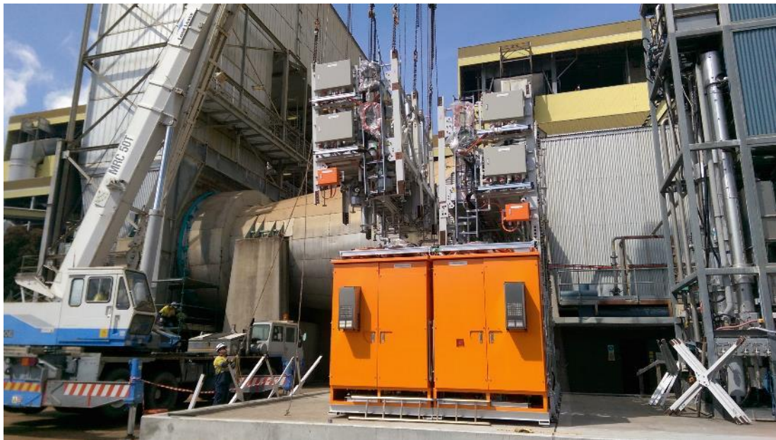
Figure 18 Fourth module being carefully lifted into position
