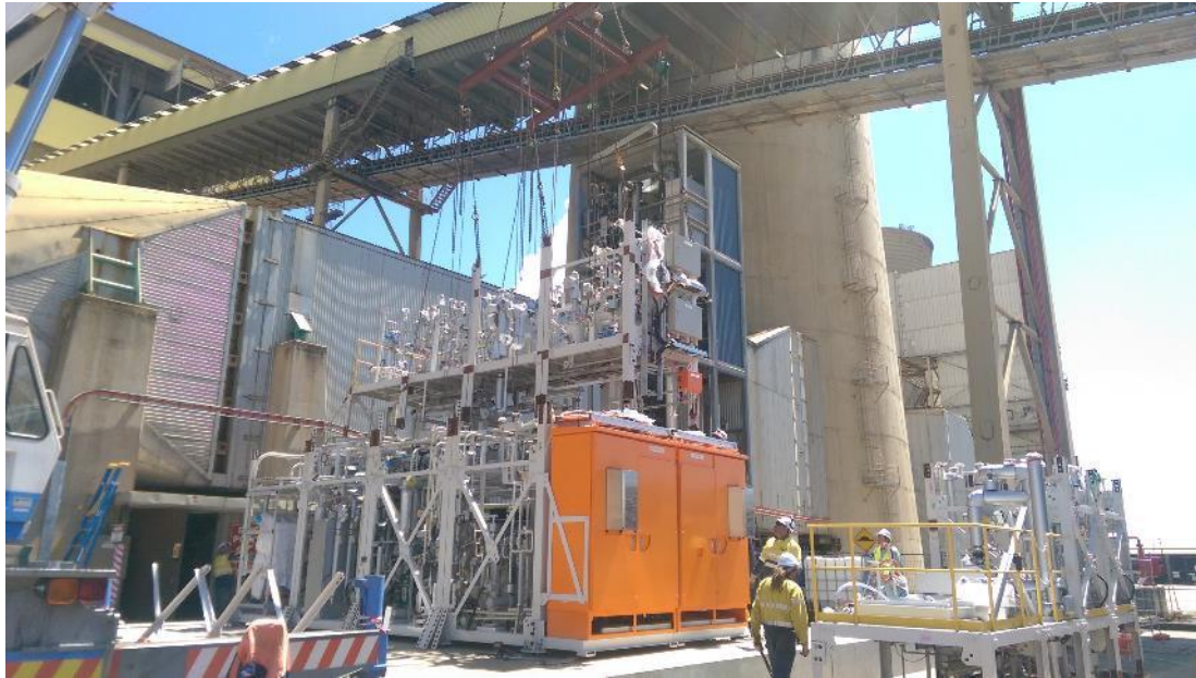
Figure 17 Third module supported by crane during installation
