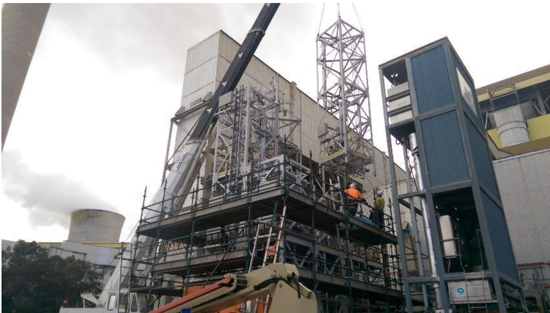
Figure 22 Eighth module installation
