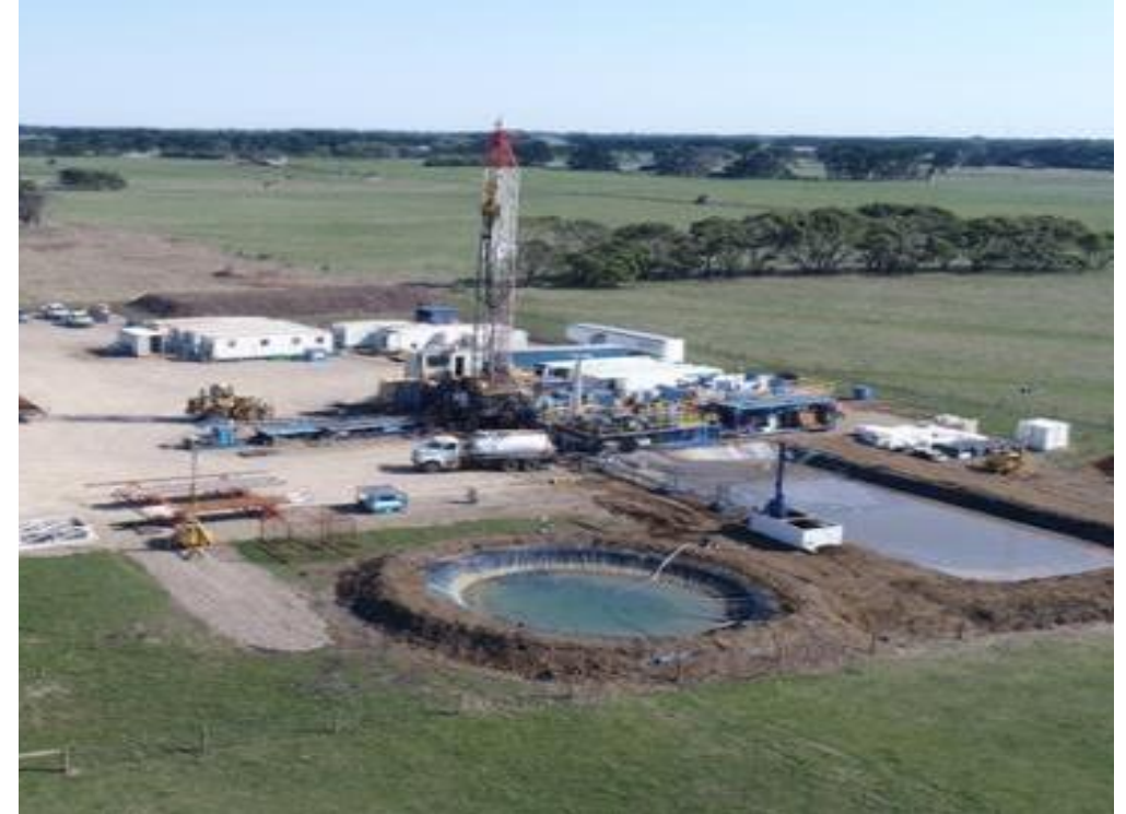
• CRC-3 drilling operations – April 2017
