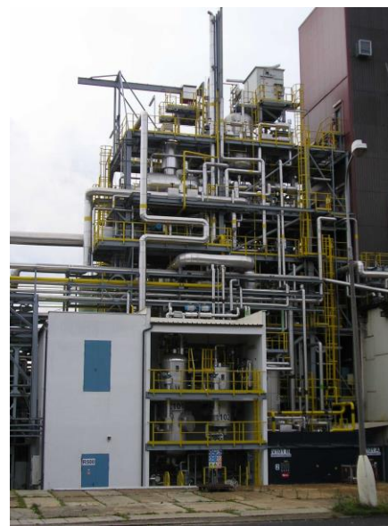
Above: Entrained flow gasifier added to the Vresova site in 2006 to gasify generator tars and other liquid by-products from the fixed bed gasifiers, courtesy of SUAS
