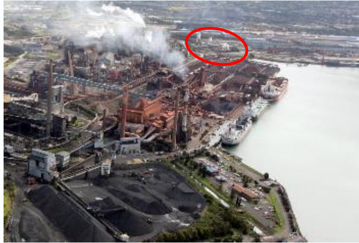
Coregas H 2 plant at Port Kembla
